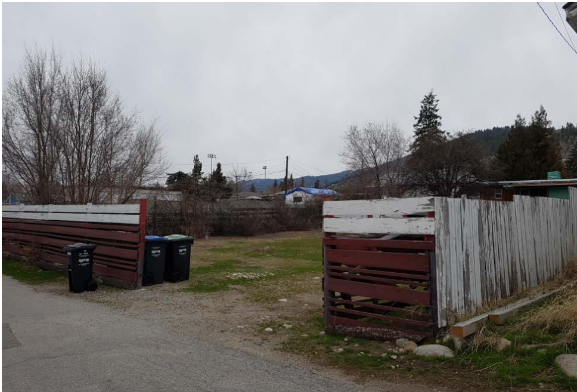
Figure 5: View from the lane
